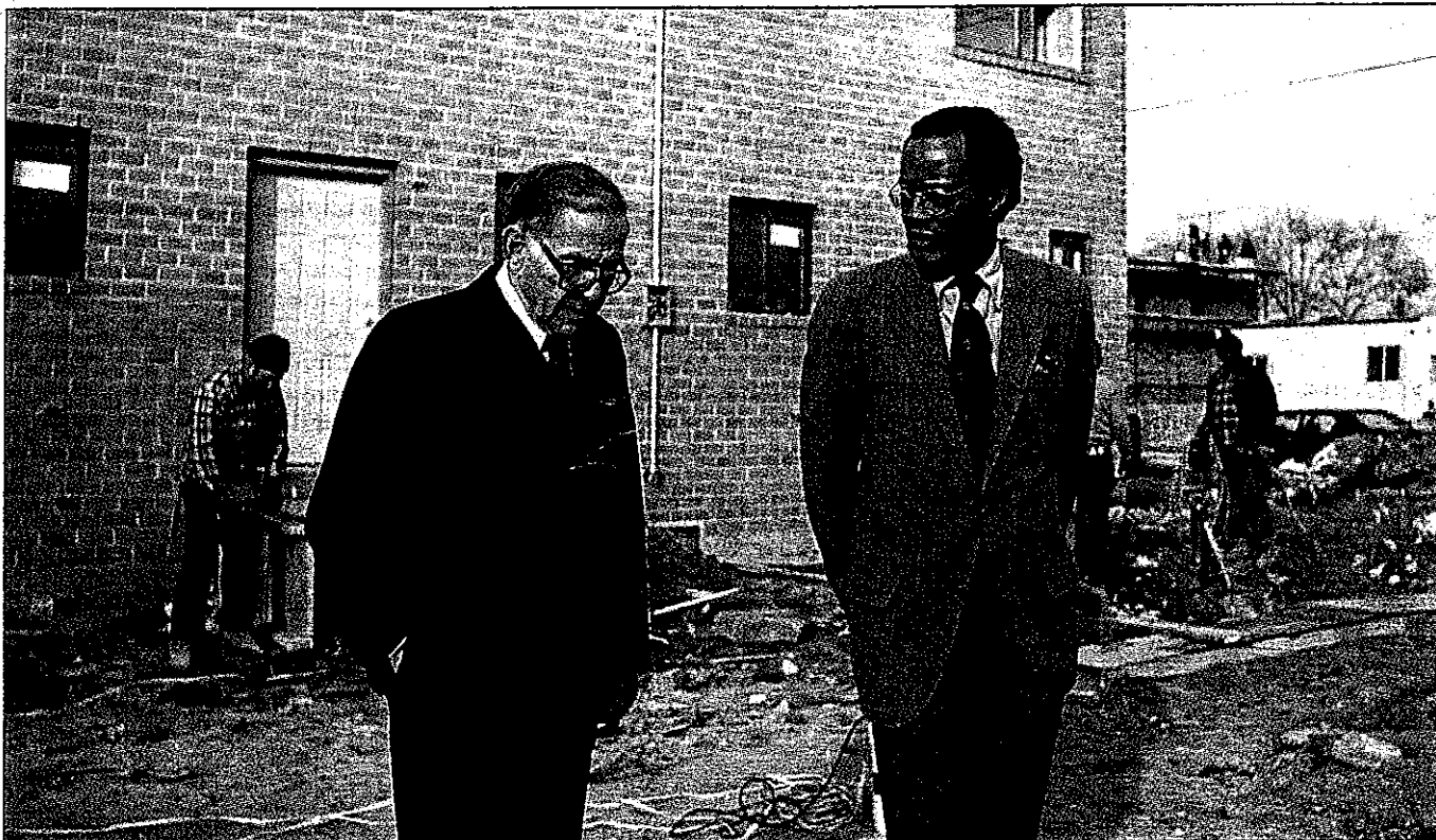
Williams and I.D. Robbins, founder of the Nehemiah Trust, survey the construction of low-income housing
